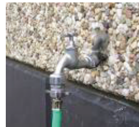
Adapter, hasp, 3/4" with air supply hose
